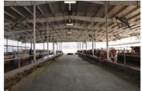
drive thru feed alley in the pack barn where cow are housed - constructed in 2006
